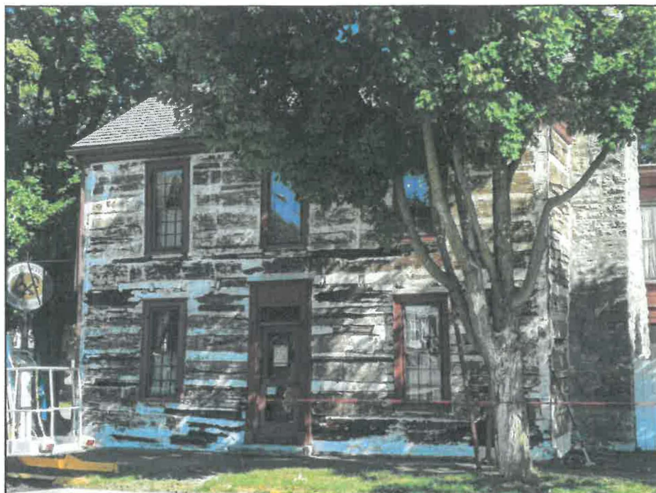
South elevation, facing Water Street.
