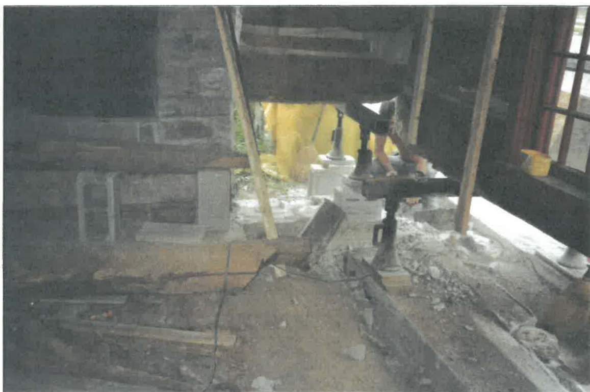
Replacement of the rotten sill log at the southeast corner of the building in 1998, view from the interior.
