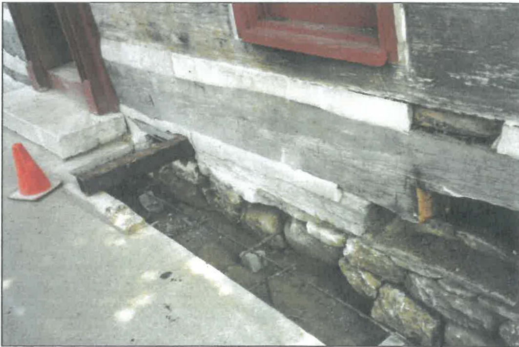
Exposing the rubble stone foundation and removal of the rotten sill log at the southeast corner of the building in 1998.
