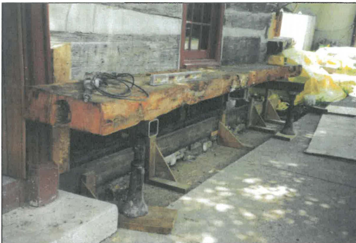
Replacement of the rotten sill log at the southeast corner of the building in 1998.
